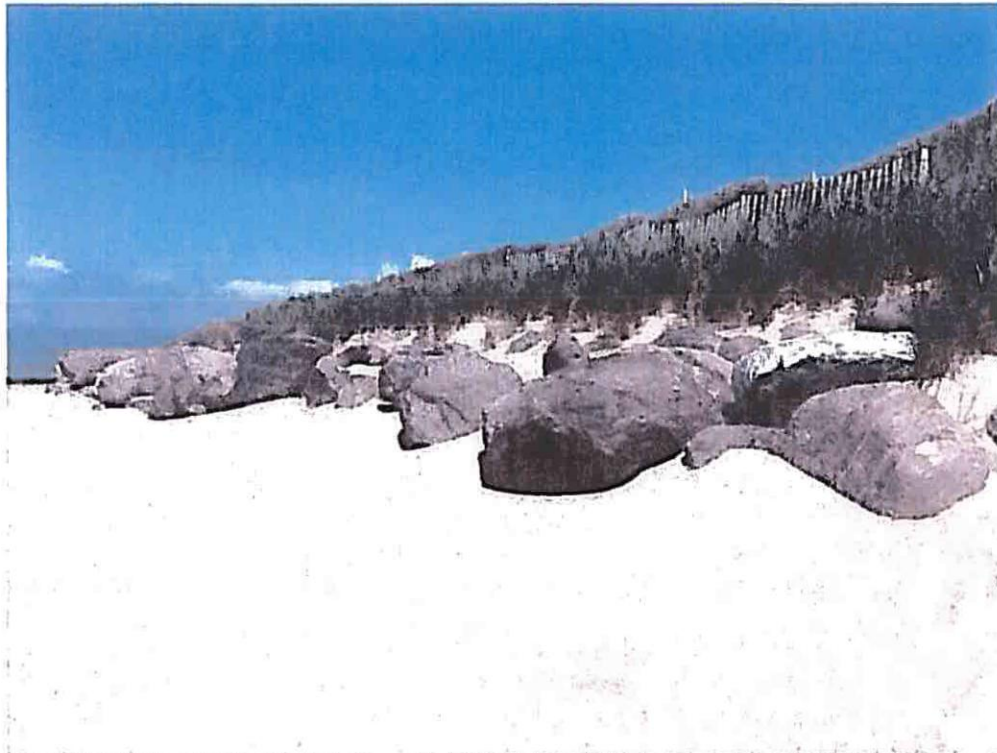
FIGURE 11: Sand fencing and rock armour protect the dunes near Dooks. Here, the system is accreting and a potential source of sediment during storms.
